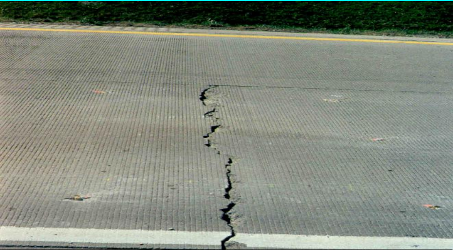
Transverse Cracking
